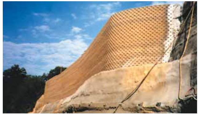
View of wall with soil nailed "bench" below.
