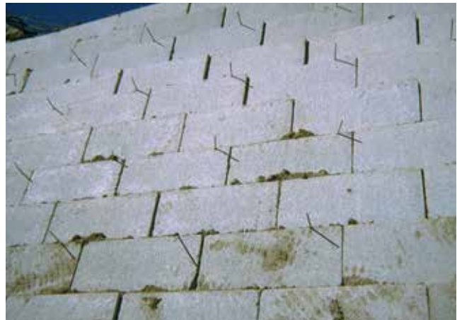
Straight face, unsplit Keystone Standard units with a 9 gauge wire provided the surface and method for attaching the rock veneer.
