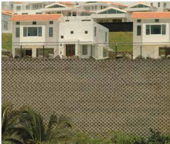
The structural integrity and flexibility of the KeySystem I wall made it efficient to design for bearing pressures of almost 10,500 psf, making it the perfect structure for the Hacienda Real soil conditions.
