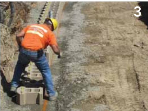
Three units are moved into place with operator guidance.
