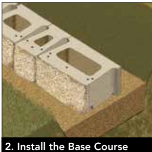
2. Install the Base Course
