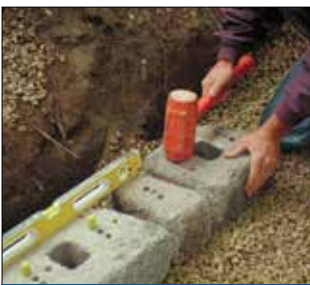
2. Install the Base Course
