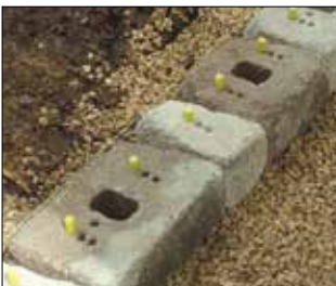
3. Insert Fiberglass Pins
