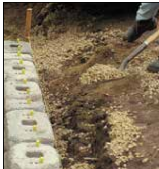
4. Install Fill & Compaction
