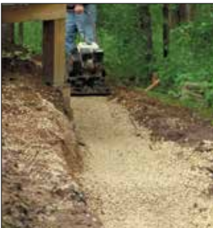
1. Prepare Base Leveling Pad
