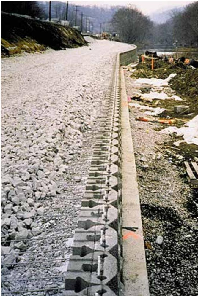
Concrete leveling pad, curved geometry & select drainable backfill.
