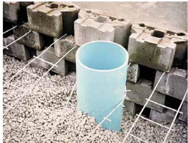
Detail at intersection of vertical post form & KeySteel reinforcement
