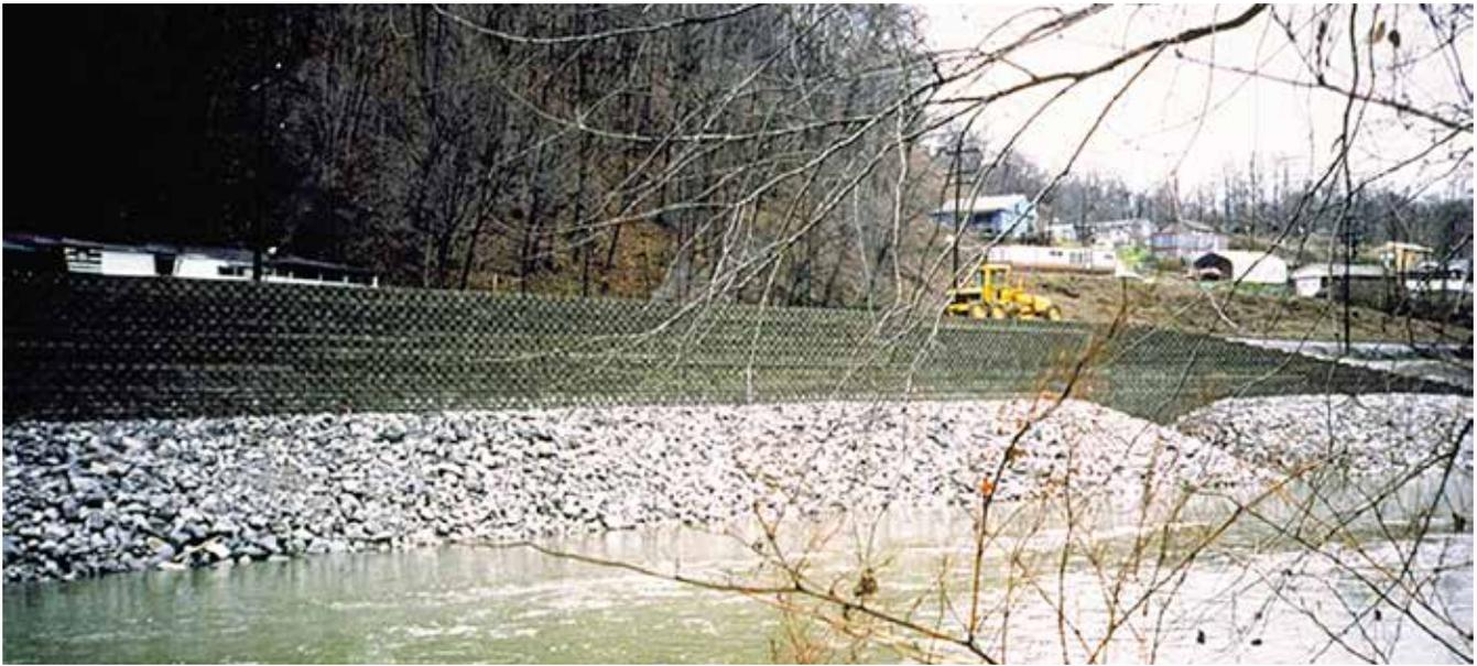
Partial wall shown with forming for additional concrete leveling pad
