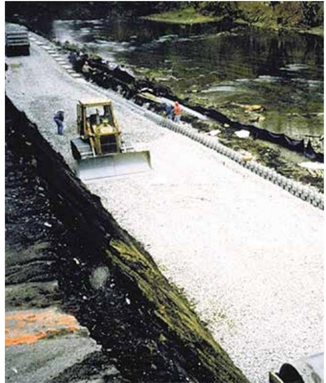
Reinforced fill zone using "select" drainable fill
