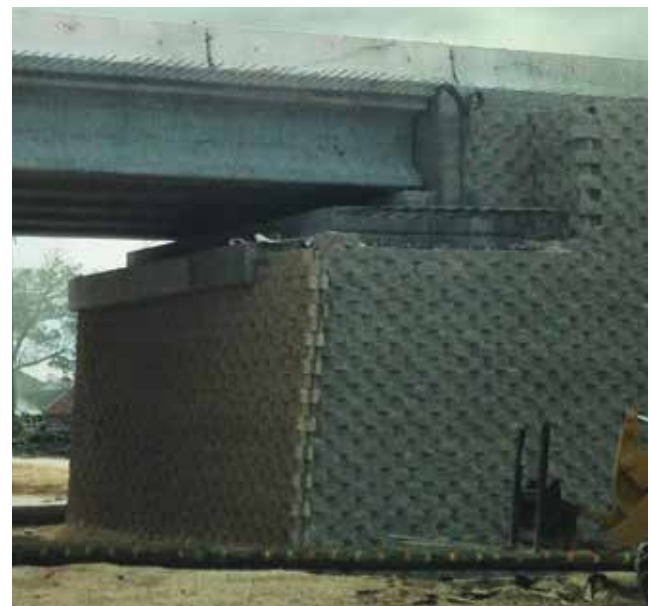
Phased Construction Temporary Wall
