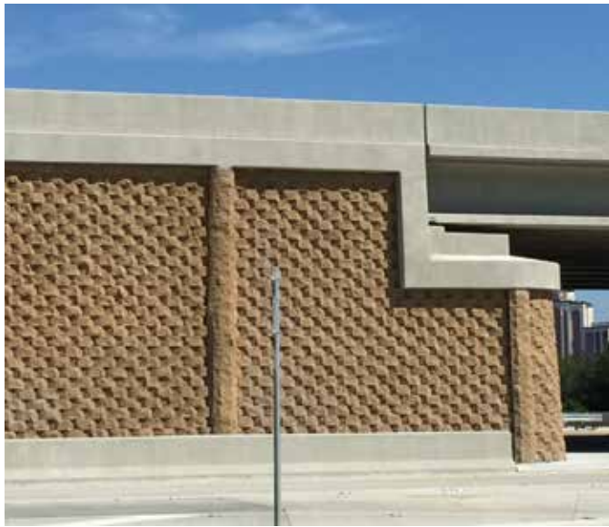
KeyGrid to KeySteel Transition Joint
